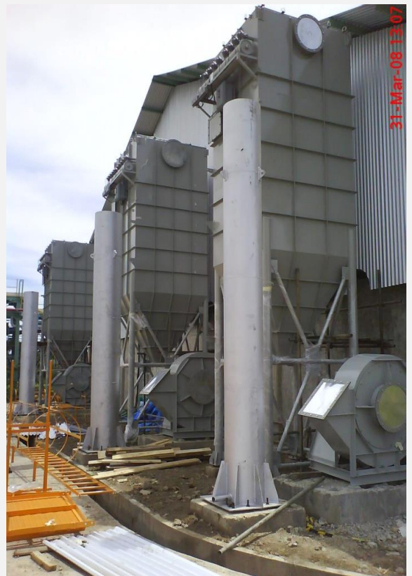
Erection Dedusting Equipment
