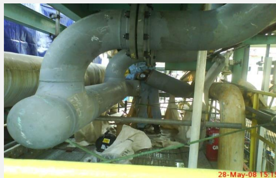
Piping Replacement Work During ASC ASDM 2008 , Work
