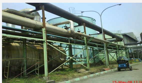
Piping Construction for Steam Line at PT. Permata Dunia
