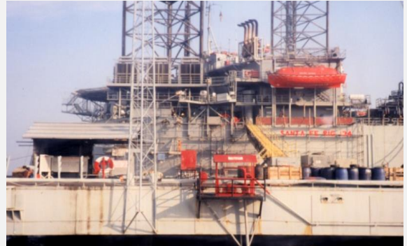
Maintenance Work for Santa Fe Rig 134 Upgrade Project
