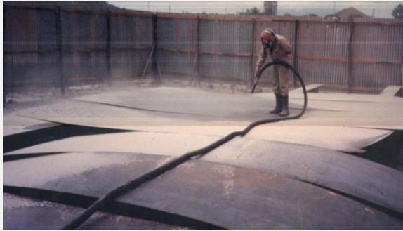
Sandblasting & Painting Work (ASC Project) from PT.
