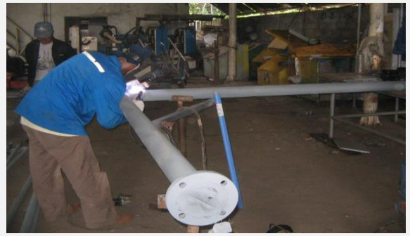
Piping Work for ASC ASDM 2007
