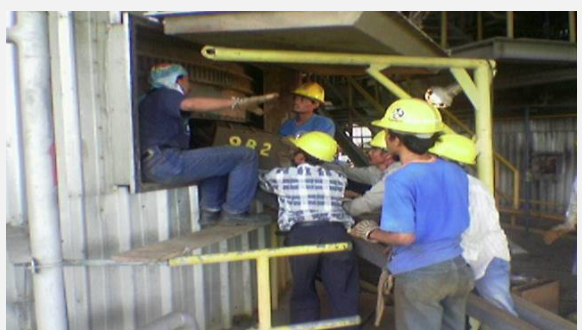
Service & Maintenance of Overhaul Boiler No.#6 from PT. Dian Swastatika Sentosa
