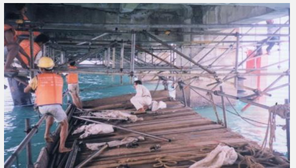
Scaffolding Work for Repair of Concrete Under Jetty at PT.
