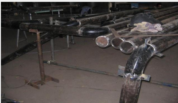
Fabrication Spool Pipe for Stack Piping
