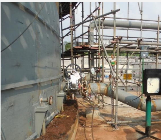
Piping Work at PT. Cabot Indonesia
