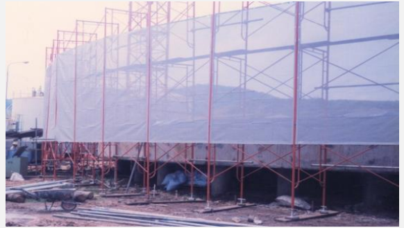
Scaffolding Work for Ethylene Storage Tank ASC Project
