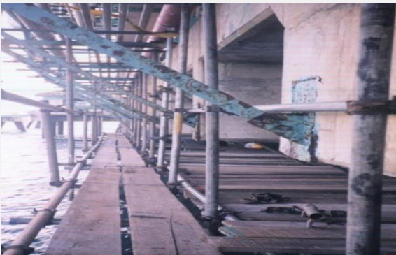
Scaffolding Work for Repair of Concrete Under Jetty at PT.
