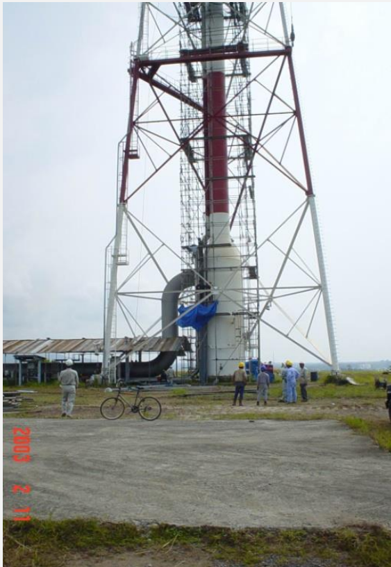
Scaffolding Work for Flare Stack Until 110 M High During PT.
