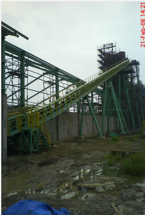
Construction for Pipe Belt Conveyor Coal Boiler Project at PT. Asahimas Chemical
