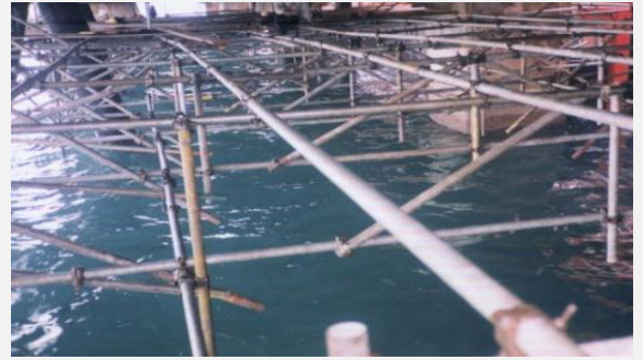
Scaffolding Work for Repair of Concrete Under Jetty at PT.
