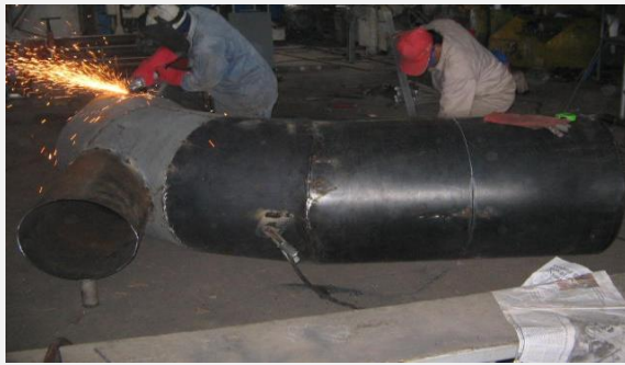
Fabrication & Painting Work for Ducting CL-1 PT. Cabot
