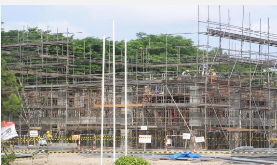
Scaffolding Work for COGEN Project PT. Cabot Indonesia
