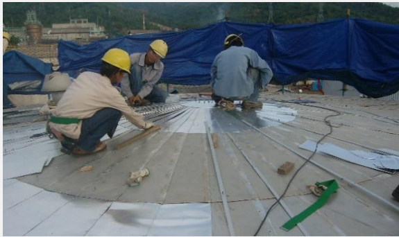
Repair Insulation Roof Tank at PT. Vopak Terminal Merak
