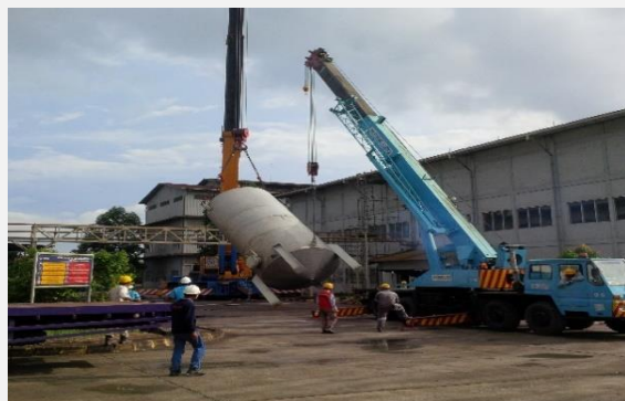
Erection of Storage Tank PT. Timah Industri
