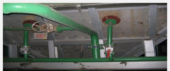
Service & Maintenance Overhaul Boiler at PT. Dian Swastatika Sentosa
