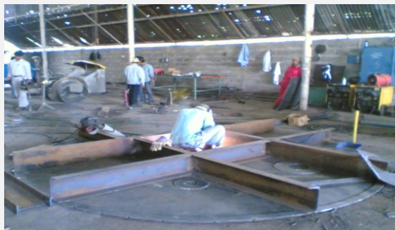
Fabrication Roof Storage Tank PT. Suprabakti Mandiri
