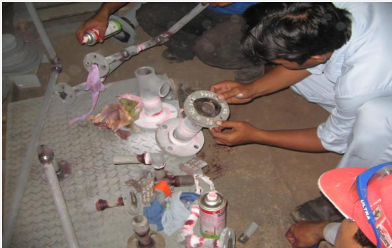
Inspection Penetrant Test by PT. Asahimas Chemical
