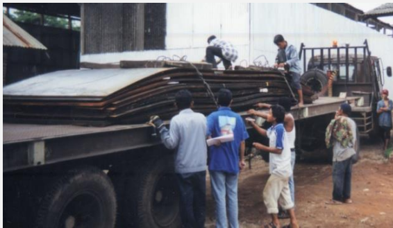
Loading Steel Plate for Cold Cutting Hommon Project from
