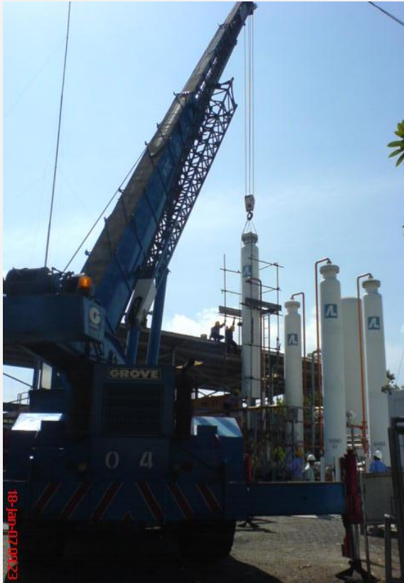
Replacement of Veseel Adsorber PT. Air Liquid Indonesia
