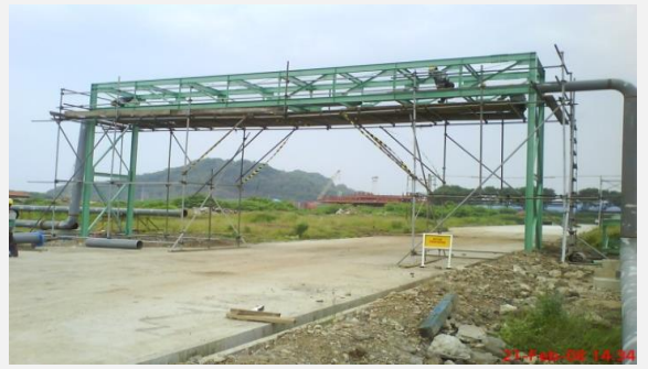
Fabrication & Installation Piperack at PT. Asahimas Chemical
