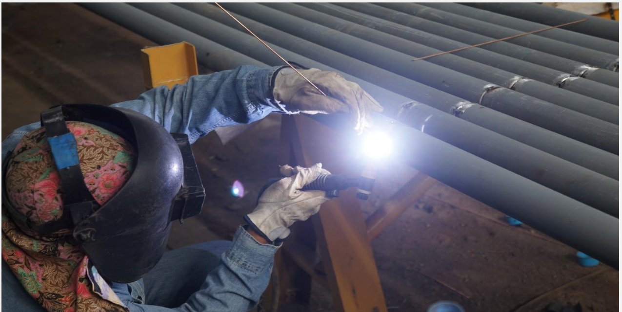
Shop Fabrication Pipe Line for OSBL Metal Piping Work of Power Plant Project at PT. Asahimas Chemical
