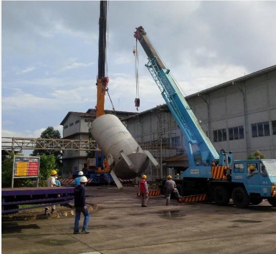
Relocate Silo Tank at PT. Timah Industri
