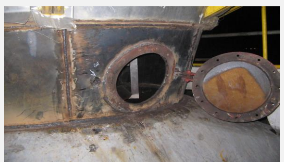
Repair Hopper During Minor Maintenance Overhaul Boiler
