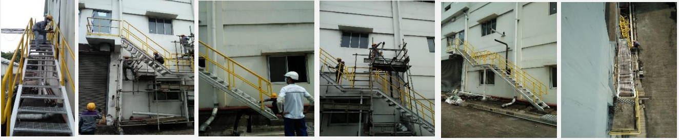
Installation Emergency Stair at PT. Tereos FKS Indonesia
