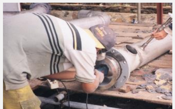
Buffing Work for Jet Pack Silo (JPS) Project at PT. Asahimas
