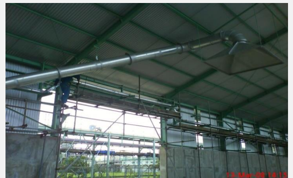
Construction Dedusting System for Coal Boiler Project
