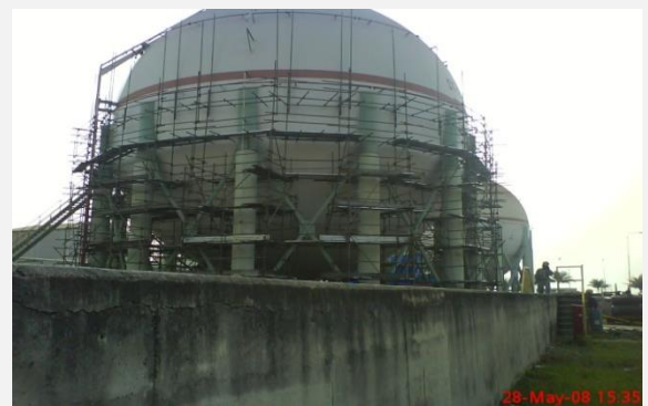
Scaffolding Work for Painting Work Ball Tank
