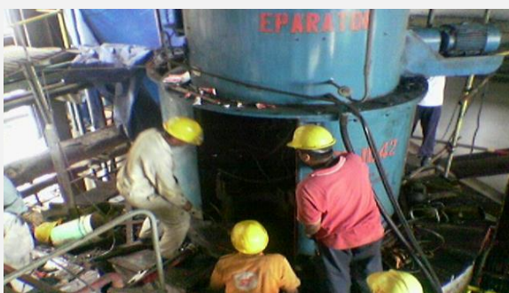
Service & Maintenance Roll Mill A.B.C. Boiler #6 from PT. Dian Swastatika Sentosa
