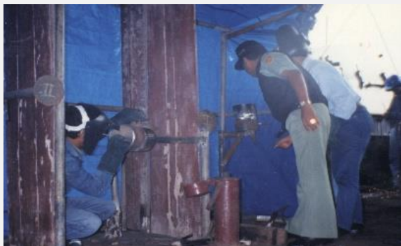
Welder Test for Santa Fe Rig 134 Upgrade Project
