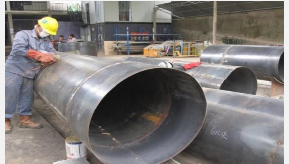
Fabrication Ducting for NGK Project Cikarang
