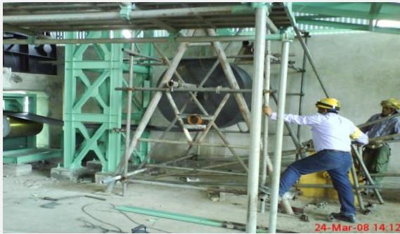
Install Belt Conveyor for Coal Boiler Project at PT. Asahimas
