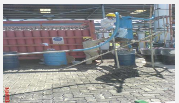
Replace Adsorber by Vacuum PT. Air Liquid Indonesia (UIC Plant)
