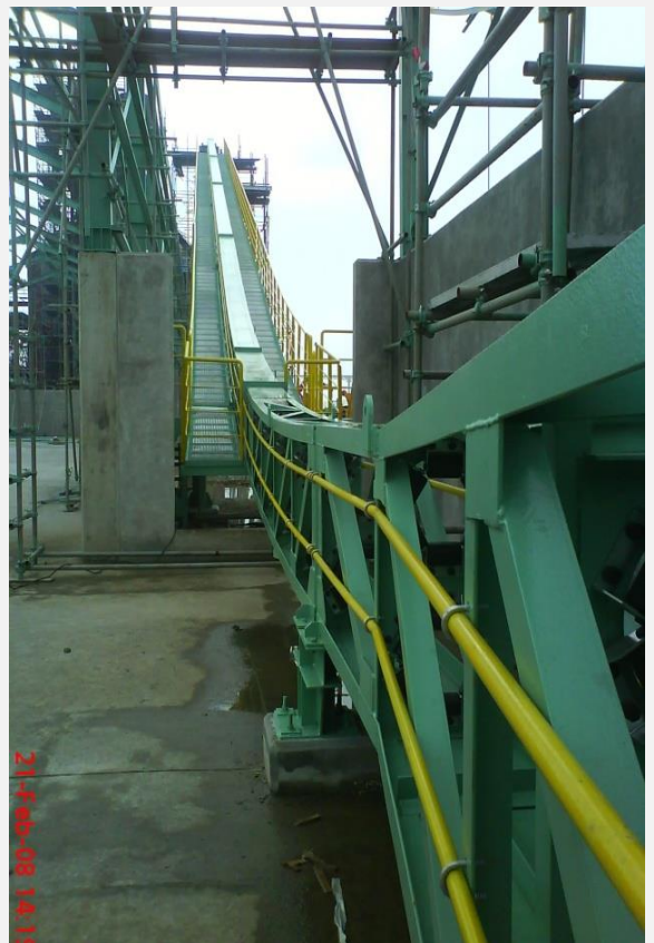
Construction for Pipe Belt Conveyor Coal Boiler Project at PT. Asahimas Chemical
