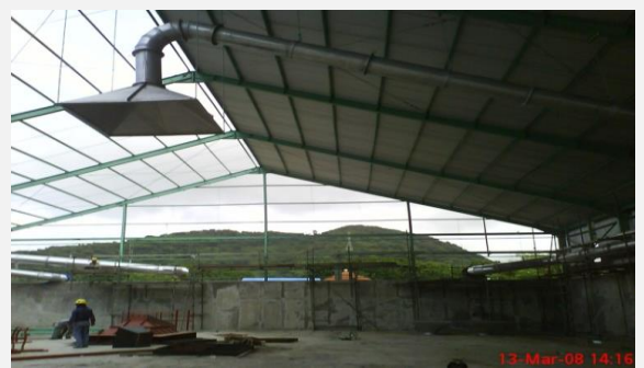
Construction Dedusting System for Coal Boiler Project
